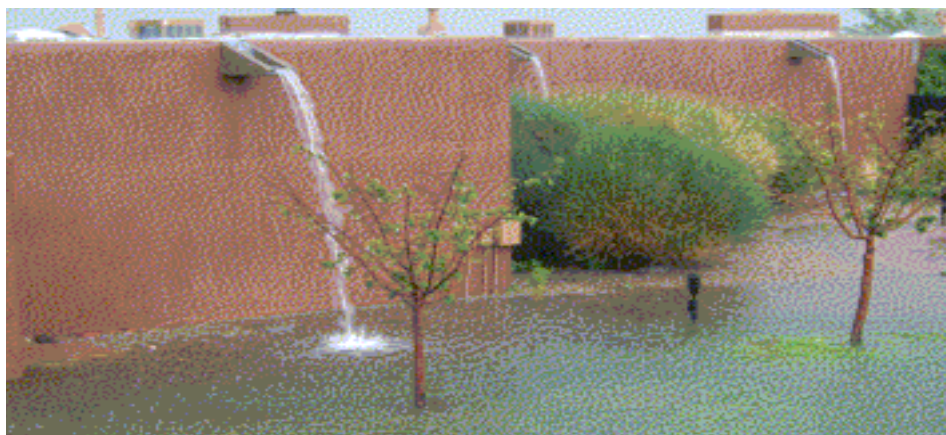
Water from canales can result in erosion and flooding if protection is not provided. Although we are in an extended drought, extreme rain events will continue to be possible. The photo shows one such event. Storms in most years do not result in such heavy runoff. Photo: Marc Hirschy
