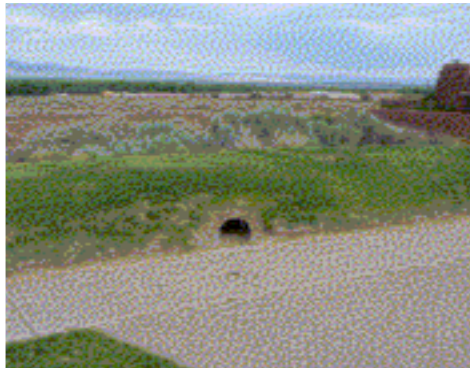
Drainage culverts have been added to berms to allow the escape of floodwater (photo below).
