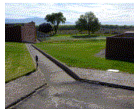
This sidewalk cleverly functions as a drainage channel through the tennis courts /pool area.
