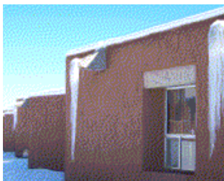
Winter drainage from roofs blocked by heavy ice dams on canales. Photo: Marc Hirschy
