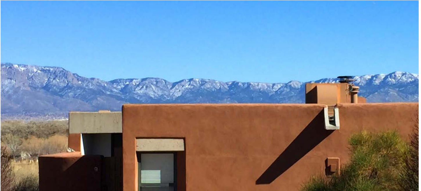
example of properly clustered roof appliances
